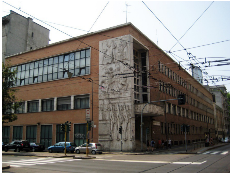
Fig. 10: Casa del Fascio by the Fabio Filzi group near to Milan Central Station with a glimpse of the Grattacielo Pirelli in the background. Photograph: Daniel Grünkranz.
